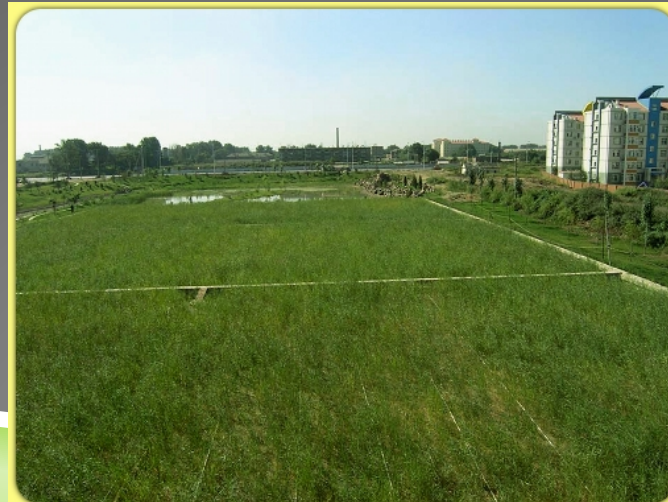
Constructed wetland, Shenyang
